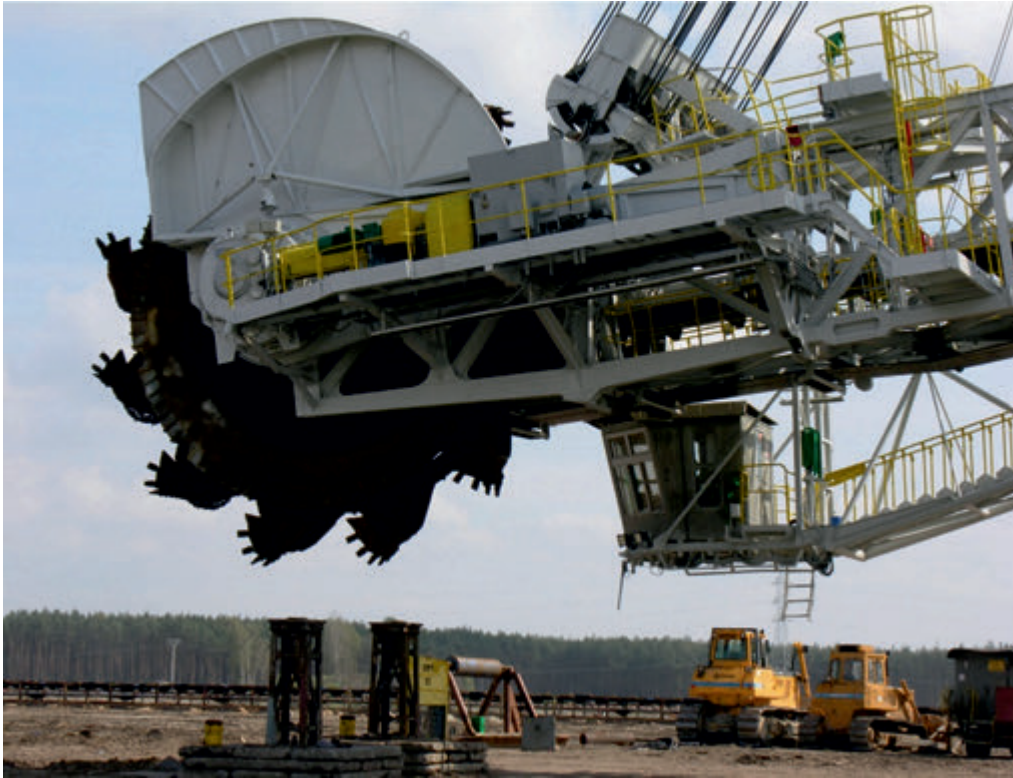
Fig. 12. Modernized drive mechanism of bucket wheel in BWE KWK 1500s at lignite open pit mine Konin
