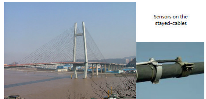
Fig. 6. The picture of bridge and experimental devices
