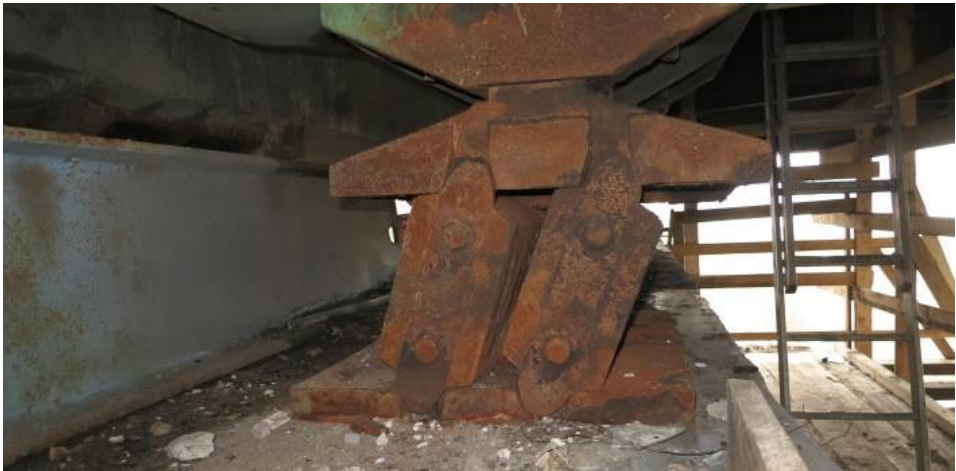
Fig. 8. Maximum permissible rotation of the bearing on the pier 13
