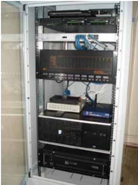
Fig.4. Hardware supervising the restricted traffic zone system in Katowice.
