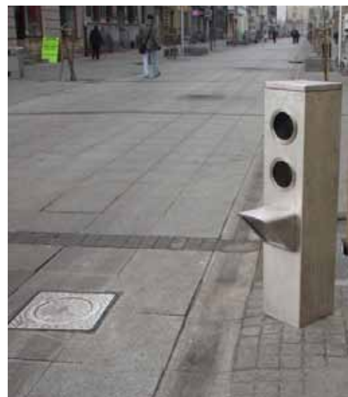
Fig.3. Pillar with built-in camera for automatic license plate recognition equipped with red-green light signaling (on the left hand side lowered hydraulic pillar on the ground level).
