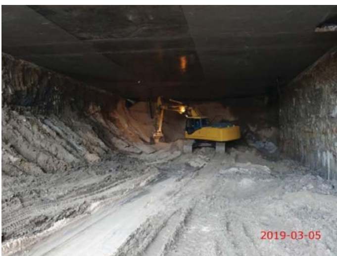
Rys. 8. Wykop pod stropem tunelu [21]
