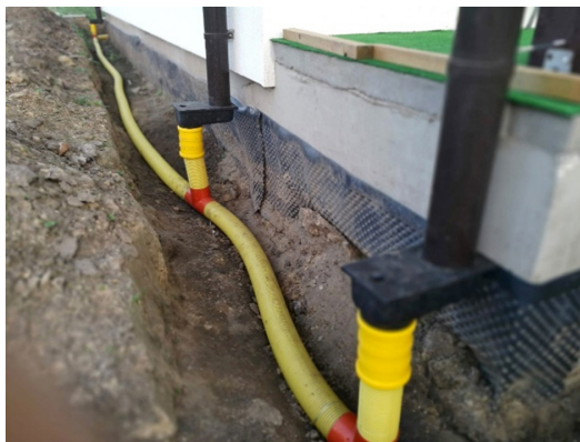
Fig. 15. Rainwater interception system;
