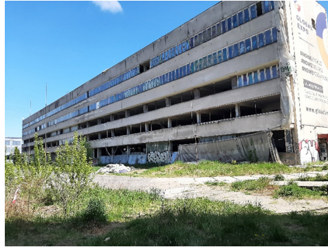
Fig. 10. GlobalExpo convention centre building on 7 May 2022; Source: own elaboration
