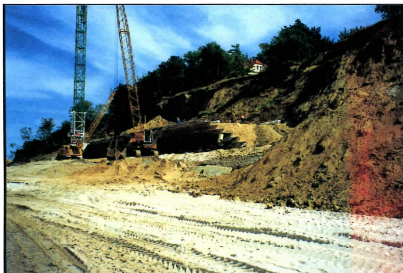
Fig. 6. Construction of block 'A'
