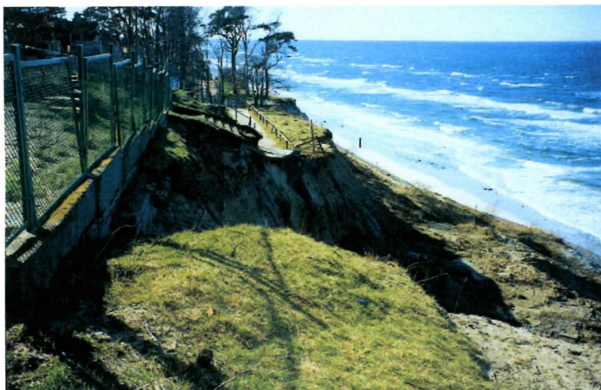
Fig. 1. Landslide in front of Villa "Mewa" – spring 1999
