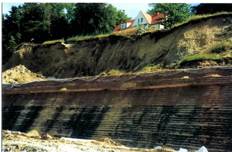
Fig. 7. Outer slope of block 'A' – the Green Terramesh system
