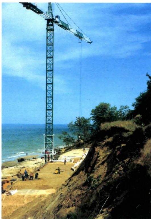
Fig. 8. Beginnings of work on block 'B'
