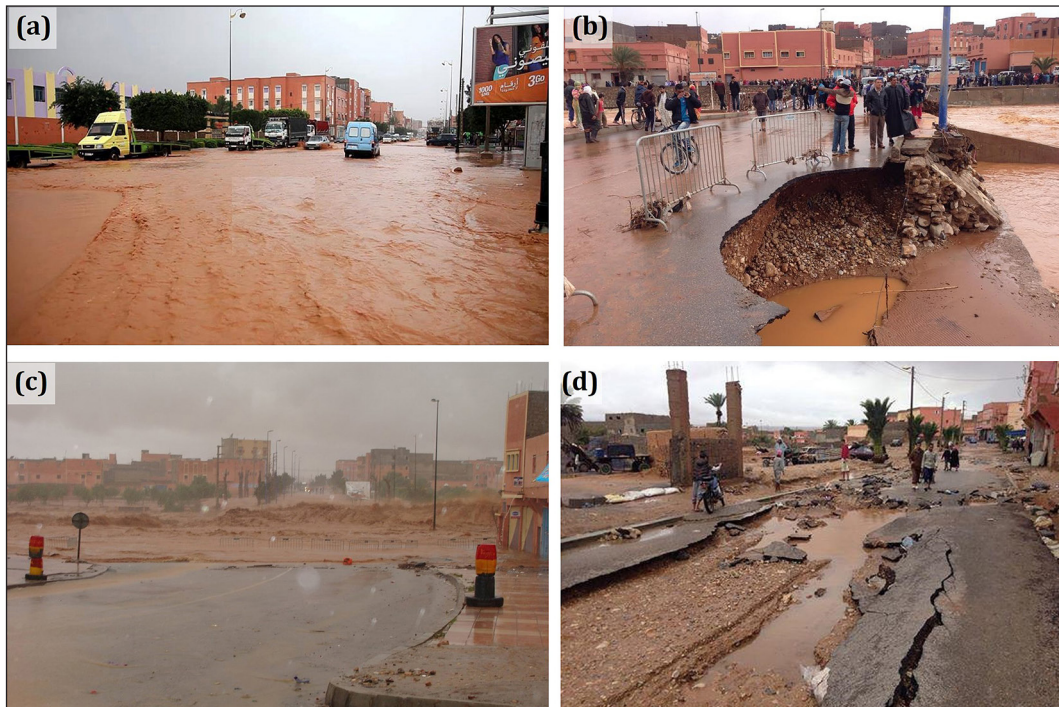
Figure 9. Photographs showing the damage caused by the floods in the Assaka watershed's urbanized areas; (a) Flooded zone at the center of Guelmim City; (b) Collapsing at the Bridge on the RN1; (c) Raising of the water level in the wadi Oum Laachar during a flood period; (d) Destruction of roadways in the Wadis neighborhoods
