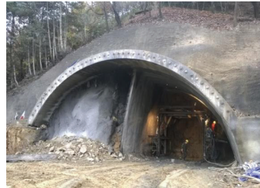
Fig. 7. Design of pipe roof in the tunnel portal Fig. 8. Construction condition in the tunnel portal
