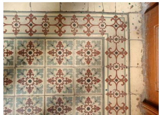
Fig. 34. Mosaic tricolor ceramic floor tiles of the Early Historicism period (44 Chuprunki Str.). Source: photo by author
