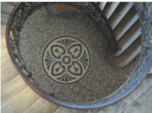
Fig. 28. Terrazzo floor with the central round element (5 Hryhorovycha Str.) Source: photo by author
