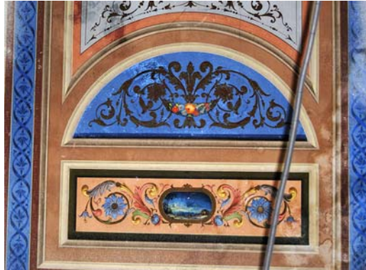
Fig. 13. Al secco murals in New Renaissance Style (arabesque, ultramarine background) on the ceiling of the staircase (4 Lysenka Str.). Source: photo by author
