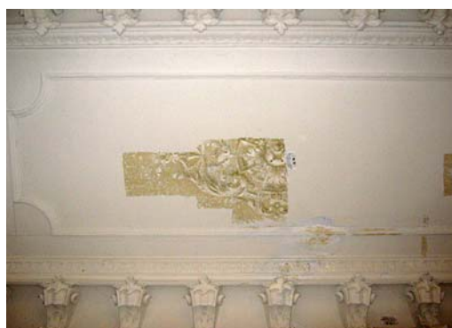
Fig. 4. The beginning of restoration of polychromy of vestibule with the sounding of grisaille rosette (school in Konyshkoho Str.). Source: photo by author
