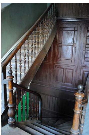
Fig. 27. Decoration with graining of the wooden surfaces in the interiors of Historicism rental houses (balustrade and paneling in 60 Hmelnytskoho Str.; apartment door in 37 Pekarska Str.). Source: photo by author
