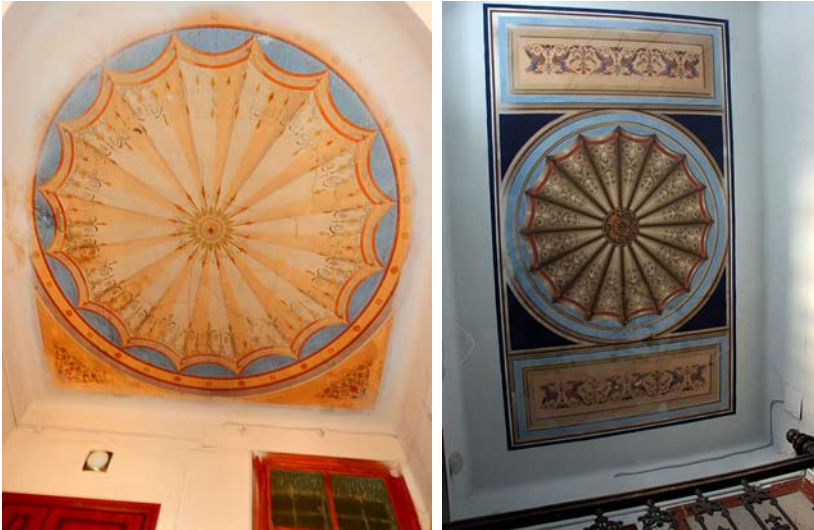
Fig. 7. Early Historicism buildings with al secco paintings in New Empire Style. The ceilings of the upper store of the staircase (Malaniuka Sq., 5 Levytskoho Str.). Source: photo by author
