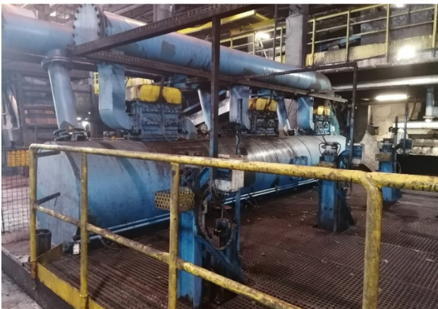
Fig. 2 OM24 jig, "Borynia-Zofiówka" Mine, Zofiówka Branch Source: [33].
