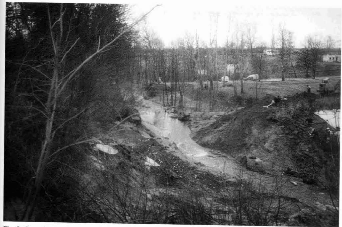
Fig. 2. General view down the river, in the foreground the broken dam
