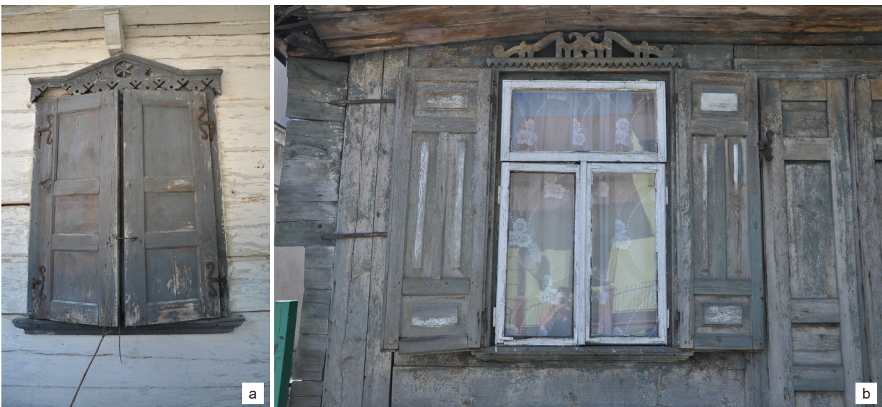
Fig. 10. A window frame with a decorative window drip and shutters in a one-story single-family house:
