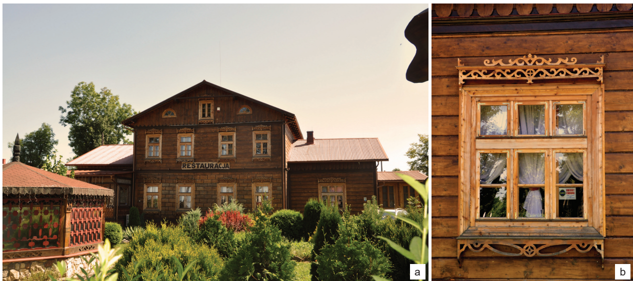
Fig. 6. A residential building from 1895, located in Słodka Street in Szczepieszyn – formerly the house of the director of the Sugar Factory Klemensów, now a restaurant: a) view from Skłodowskiej Street, b) detail of the window (photo by E. Pol, 2013)
