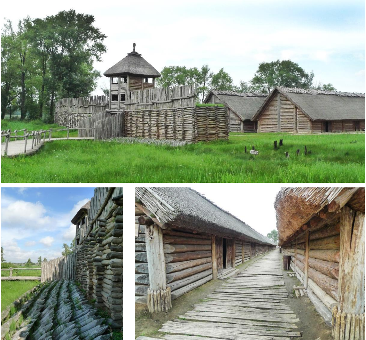
Fig. 4-6. Biskupin – reconstruction of a fragment of the wooden gord with elements of defensive and residential structures. Source: authors photographs, 2010
