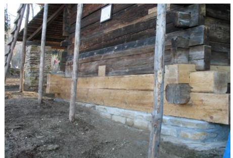
Fig. 27-30. Orthodox church in Piątkowa – left: conservation design (author: Jan Kurek), right: the building during the replacement of base plates and shingle roofing. Source: author's archive
