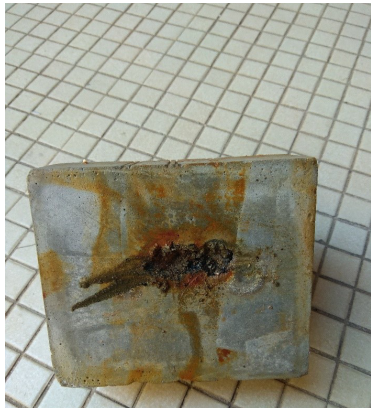
Fig. 2. Bottom view of the concrete sample.
