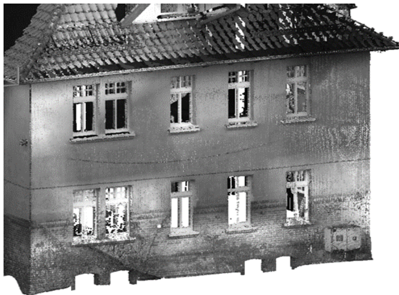
Fig. 1. A point cloud of the south-eastern elevation of a building overlaid with digital photos (own photo)
