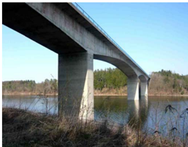
Fig. 3. The Bridge near Brzotice
