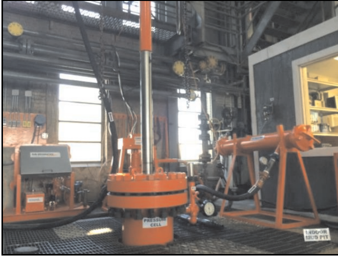
Fig. 2. TUDRP Rig. Drill floor: Rig lower level
