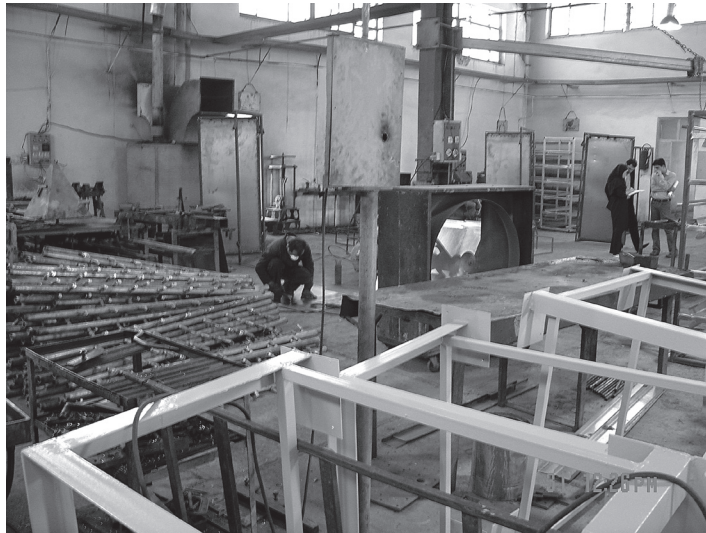
Figure 1. Worksite before improvement: poor posture, air pollution due to welding, no general ventilation.
