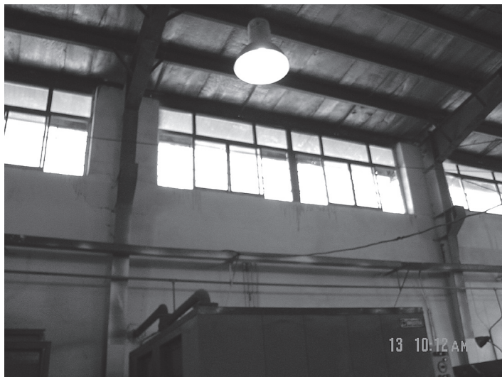
Figure 9. Worksite after improvement: light walls, improved lighting conditions and workplace atmosphere; clean windows and well-maintained light sources help to increase lighting.
