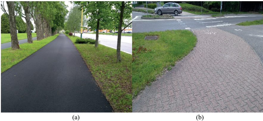
Fig. 8. A brand new paved cycletrack: (a) new surface, (b) segments with crossing and paving
