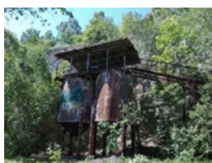
Fig. 7. Vertical lime furnaces in the pit (Source: Z. Łacny)
