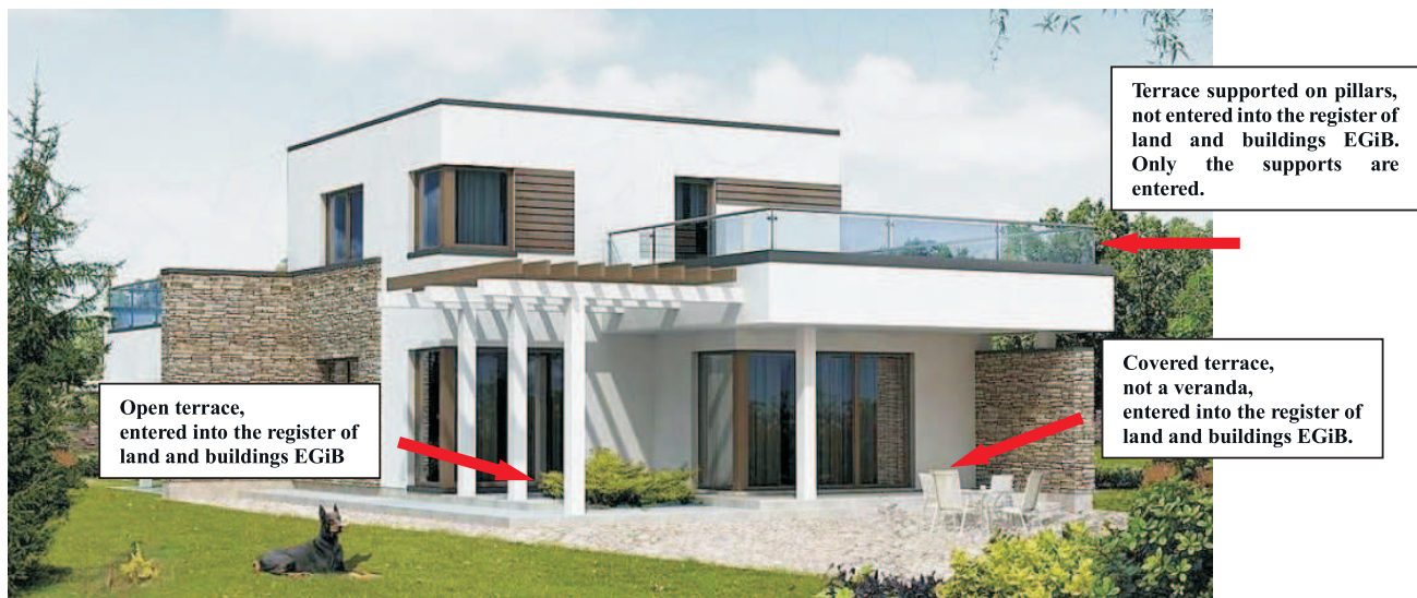
Figure 3. Terrace or Veranda? (Source: photograph of a building from the training materials of the Society of Polish Geodetic Surveyors)
