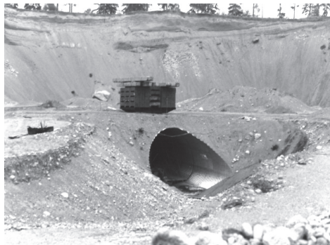
Figure 1. Enköping pipe arch, loading to failure test
