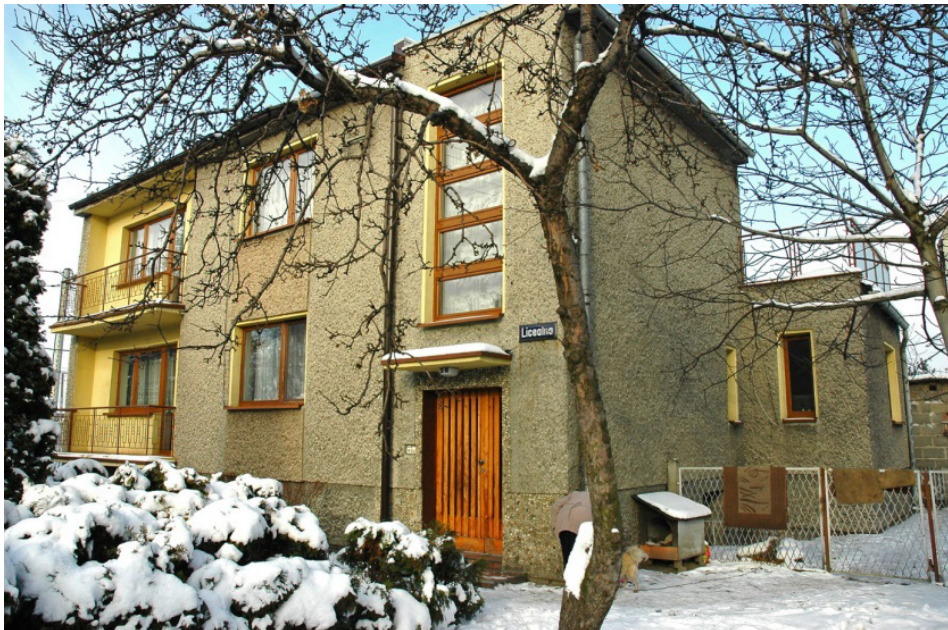
Fig. 1. View of the building from the south-east. Source: author
