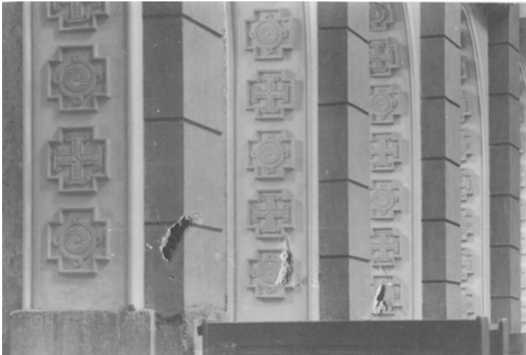
Fig. 3. Prefabricated ornaments in the church in Radom, photo from the archives of the Pieńkowski family, undated
