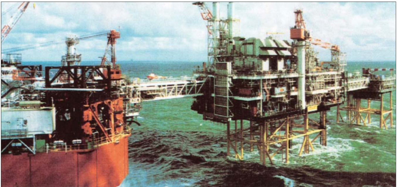
Fig. 5. Offshore platforms with connecting bridges [10]
