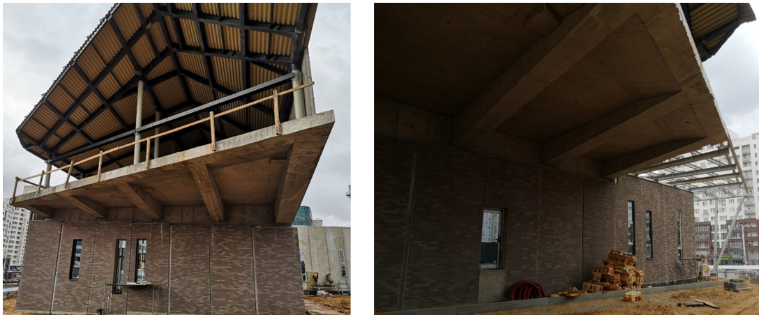
Figure 4. Sections 2, 3 – Post-tensioned monolithic cantilever sections
