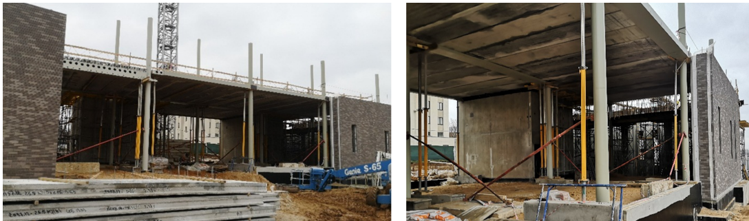
Figure 5. Section 4 – Composite steel-concrete structure
