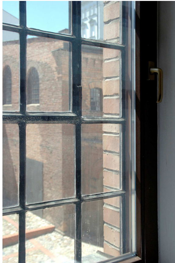
Fig. 5. Example of the installation of an additional window. Ludwig Geyer's "Biała Fabryka" (now Central Museum of Textiles), Łódź. Photo by A. Kurzac.
