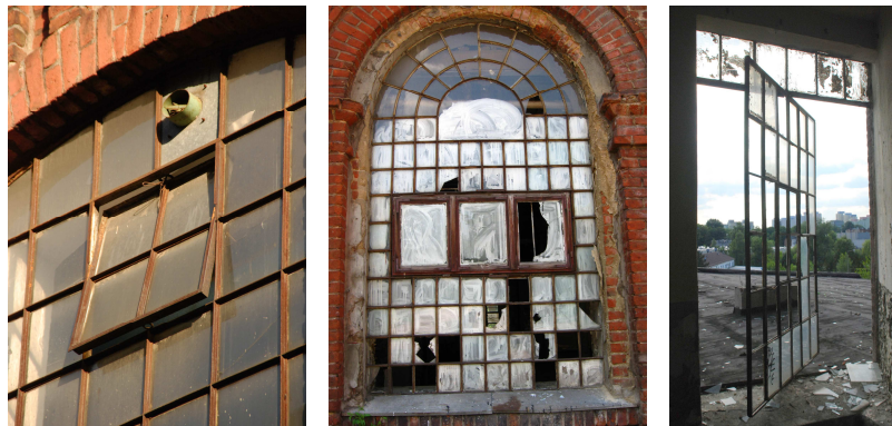
Fig. 3. Various types of hinged frames used in industrial windows. From left: Scheibler's factory, Kretschmer's spinning factory, Geyer's weaving factory. Photo by A. Kurzac
