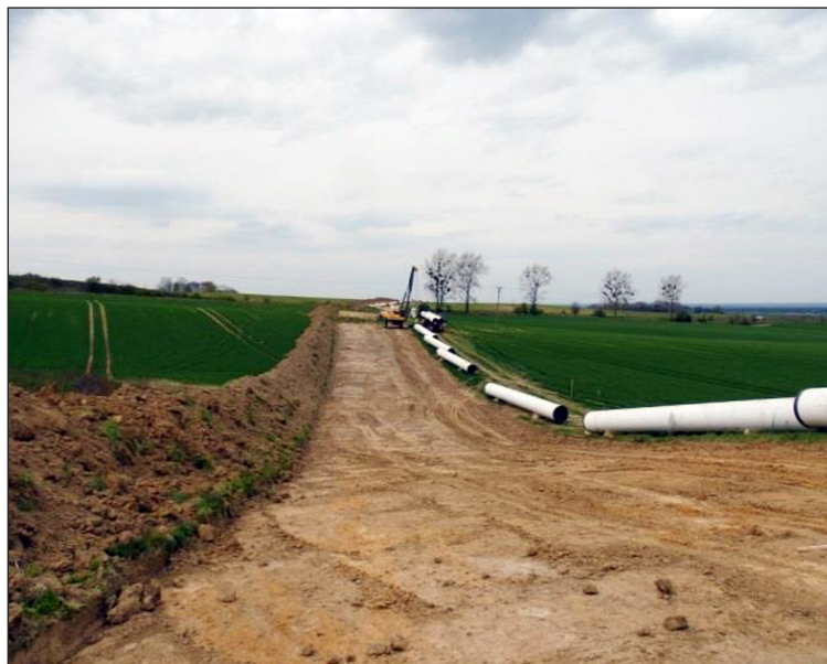
Figure 3. Image after the implementation of linear infrastructure
