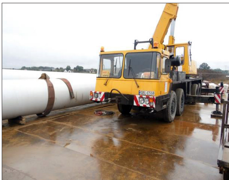
Figure 1. Application of steel plates at the construction stage
