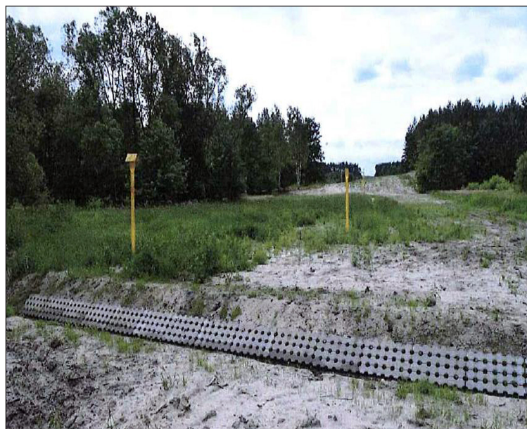
Figure 4. Image after the implementation of linear infrastructure
