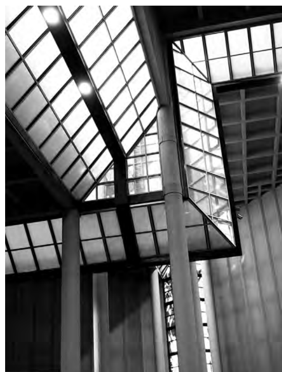
Fig. 13. Church of Saint Queen Jadwiga in Cracow, 1978–1988, project by Romuald Loegler, Jacek Czekaj; perspective interior view of the Fireflies dissecting reinforced concrete walls
