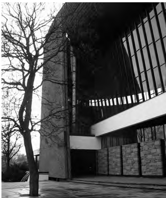
Fig. 7. Church "Arka Pana" in Cracow – Nowa Huta; 1967–1977, project by Wojciech Pietrzyk; Call one of the architectural concrete and glass exterior walls, the view from the outside – from the north
