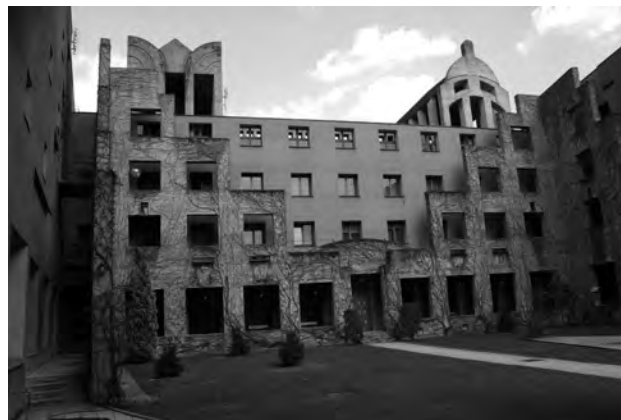
Fig. 2. The sacral center Resurrectionis XX. Zmartwychwstańców in Cracow, 1985–1993, project by Dariusz Kozłowski, Waclaw Stefański, Maria Misiągiewicz; view of the facade of the building seminar from inner courtyard
