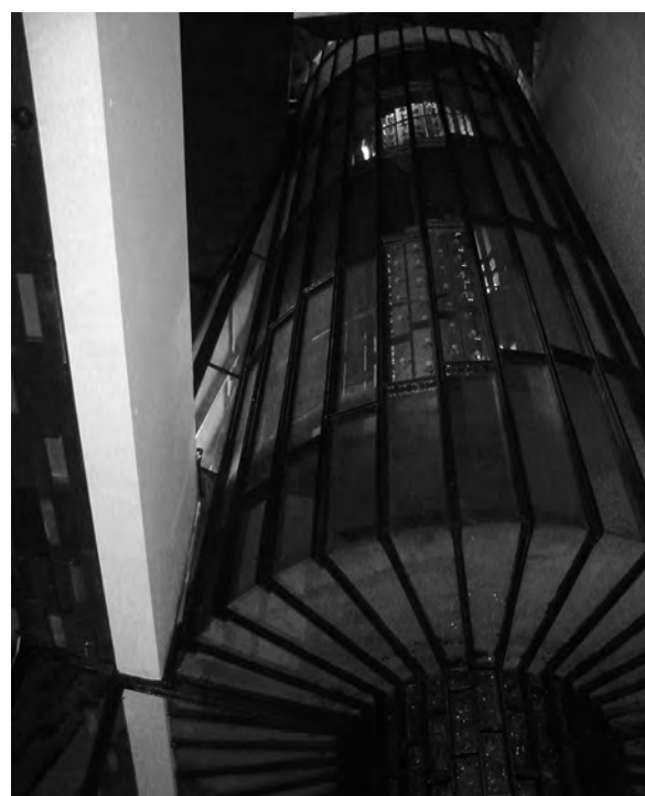
Fig. 10. Church "Arka Pana" in Cracow – Nowa Huta; 1967–1977, project by Wojciech Pietrzyk; combination of glass with concrete, cover the stairs leading to the roof, the view from the inside
