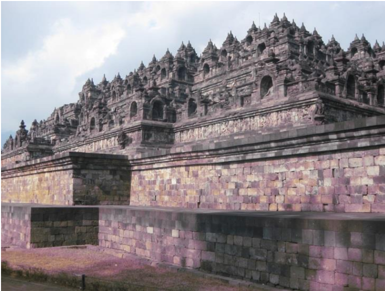
Fig. 1. Borobudur Temple, Indonesia; a photo taken from the level of the base encasement of the temple, source: author's archive, 2018
