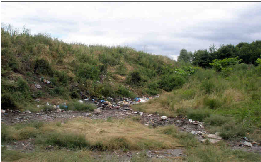
Fig. 3. The landfill slope [10]
