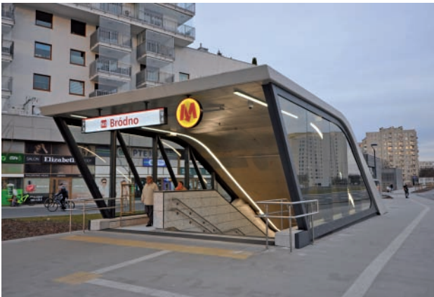
Fig. 9. The entrance to the Bródno station (18/03/2023) [photo M. Graff]
