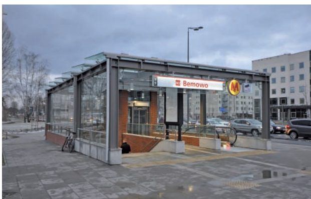
Fig. 19. The entrance to the Bemowo station (11/03/2023) [photo M. Graff]
