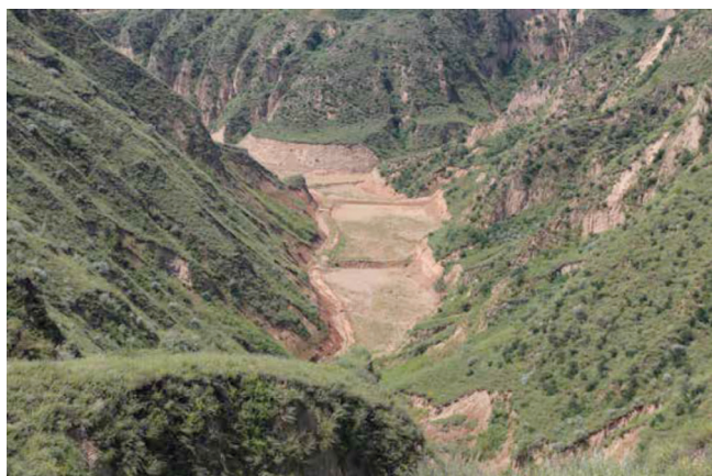
Fig. 13. Check-dam built during the Great Cultural Revolution.
