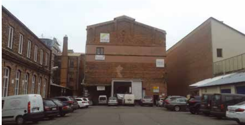
Fig. 1. The front elevation of the building in its existing condition; source: author
