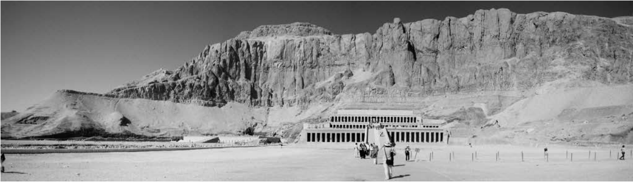
Fig. 15 – Example of long pathway towards the building: Mortuary Temple of Queen Hatshepsut, west bank of the Nile near the valley of the Kings in Egypt ; photo: Benjamin Franck
