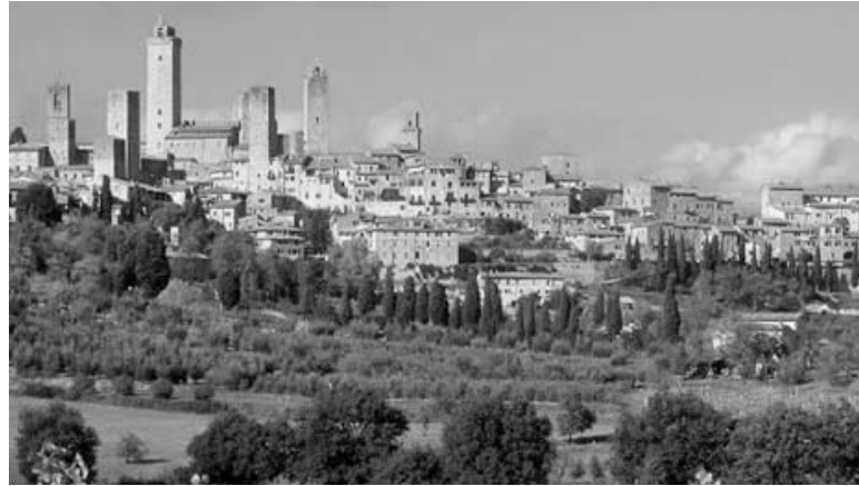
Fig. 17 – Example of status architecture: city of San Gimignano, Italy: multiple medieval towers belonged to powerful families of XI-XIII centuries, competing for status and reputation; photo: Associazione Pro Loco San Gimignano
