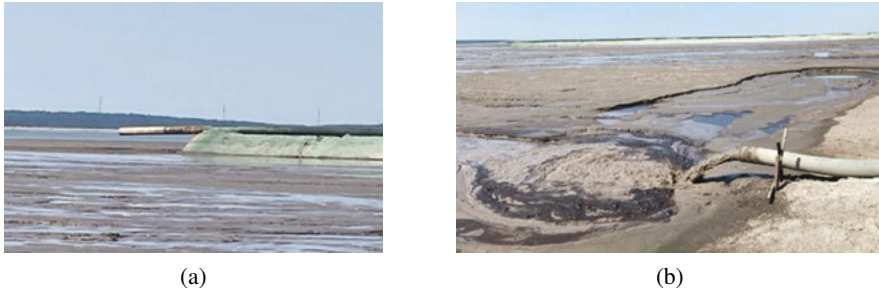
Fig. 2. Slurry deposition (a) pier, discharge point; (b) spigotting onto the beach
