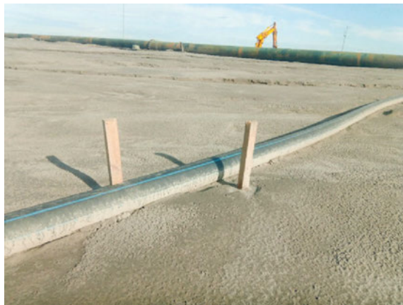
Fig. 10. Stand for the test floating pipes after spigotting
