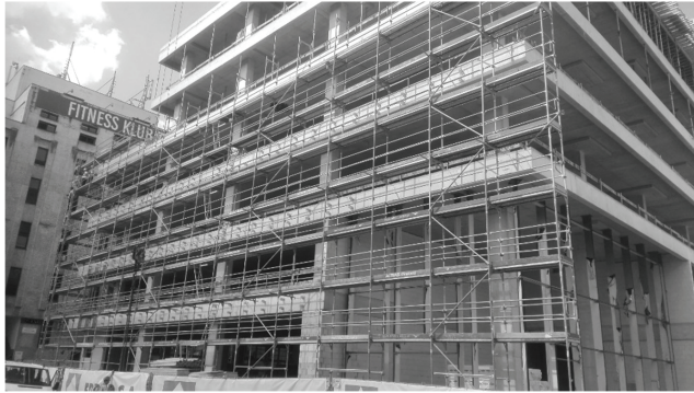
Fig. 1. Analysed full-scale façade scaffolding.
