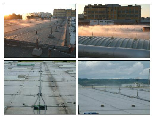
Fig. 1. Evaporative roof cooling system
