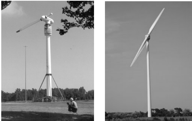
Fig. 4. Wind power stations one and two blade propeller [9, 10]
