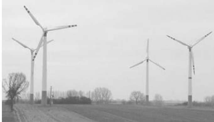
Fig. 3. Three blade propeller wind power stations of the horizontal axis installed on the bank of the backwater Jeziorsko, province łódzkie
