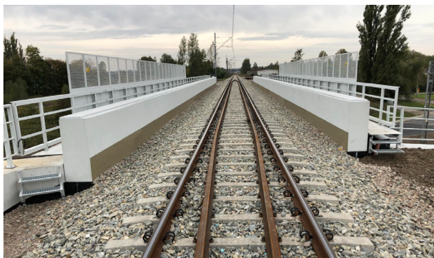
Figure 9: Bridge in Dąbrowa Górnicza after erection. Source: Nowak Mosty.
