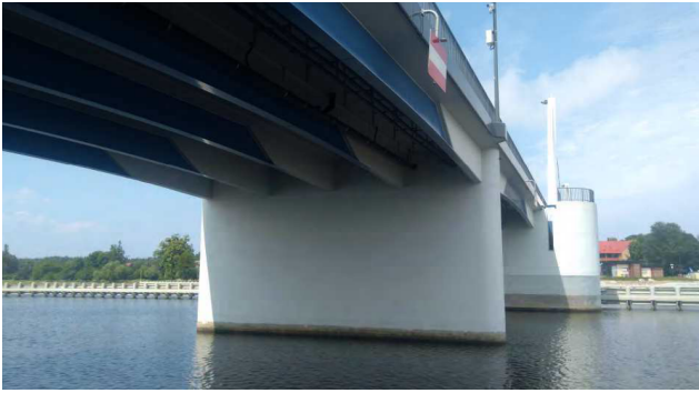
Figure 5: Hybrid beams of Sobieszewo bridge [4, 6].
