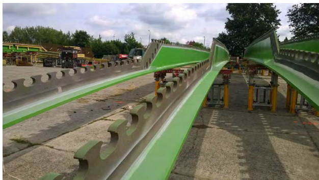
Figure 3: Steel T-sections of Elbląg bridge. High T-sections for mid-span regions, low T-sections for internal support regions [4].
