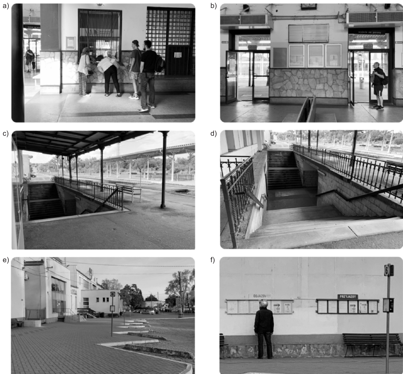
Fig. 7. Nysa Multimodal Centre – current status 07.2019: a) railway station (ticket office), b) railway station (passenger information), c) railway station (platform standard), d) railway station (access to platform), e) bus station (main entrance, departure points), f) bus station (passenger information) [authors' resources]
