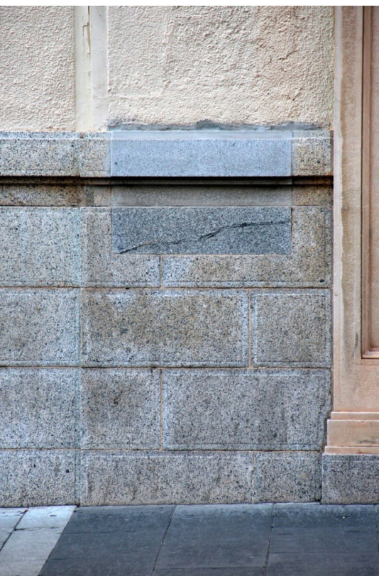
Fig. 2. The unsightly effect of compensation for the loss of with incorrectly chosen material (photo: authors' archive)
