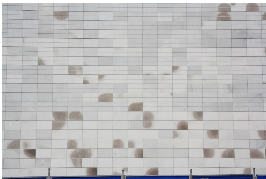
Fig. 1. Discoloration of stone as a reaction to atmospheric conditions (photo: authors' archive)
