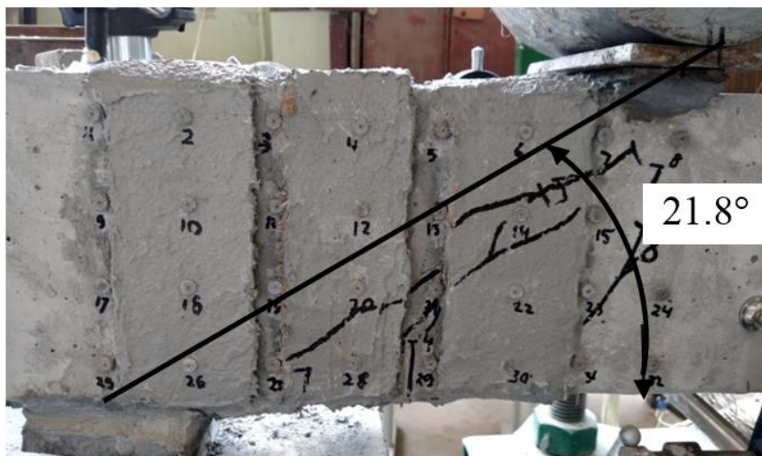
Fig. 3. The tilt angle of compressed element in strengthened sample
