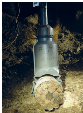
Fig. 10. ReBar Cutter™ fitting on a ∅ 55mm steel balance line
