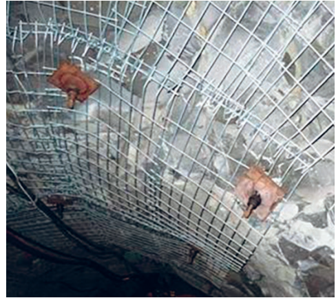
Fig. 4. Anchor housing reinforced with mesh Source: [5].
