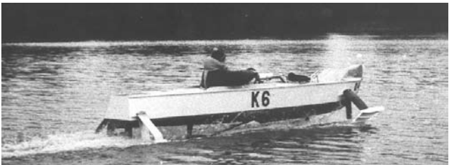
Fig. 5. The K-6 hydrofoil during tests on Jeziorak Lake.
