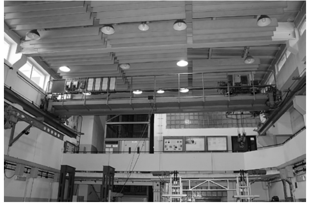
Fig. 8. The laboratory overhead crane
