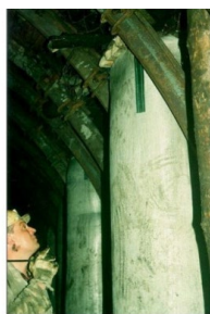
a. concrete protection pillar in adit
