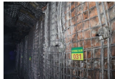
b. The artificial pillar has been completed
