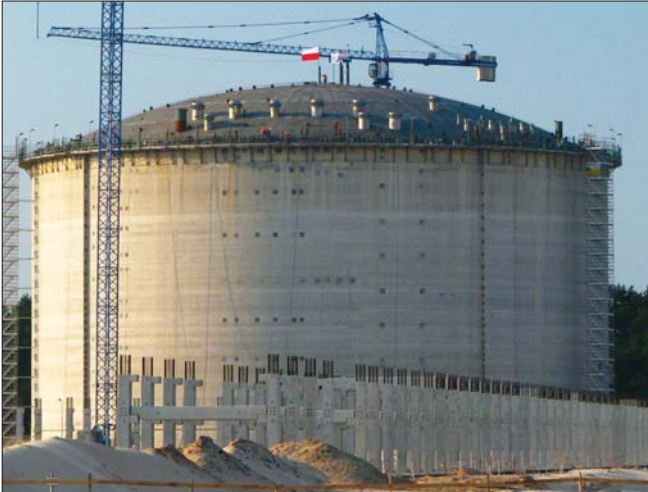
Fig. 1. View of the tank during its construction
