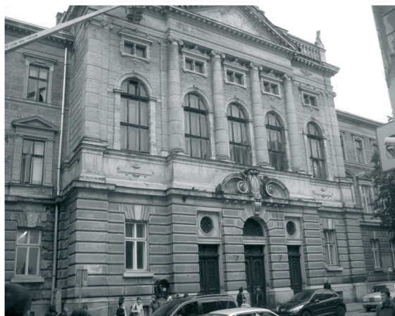
Fig. 3. The elevation of former “Palace of Justice”, built with using Roman cement. The architects: Franz Skowron and Jan Zawieyski, project 1891. Foto M.Bevz, 2011.
